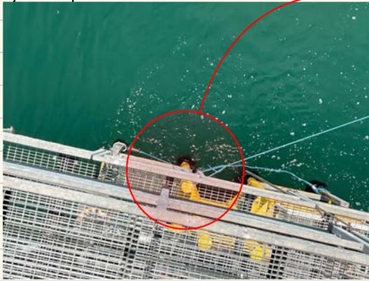
→ Looking at the level oscillations around the tower's columns is a good strategy to estimate the wave height.
